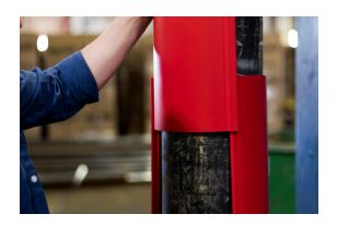
**Step #4:** Once in place, slowly interlock the final piece with the two-piece panel around the column, making sure that both sides are interlocked before sliding all the way down to the ground.
