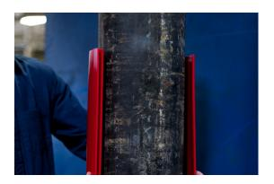
**Step #3:** Once interlocked and even, place the two-piece panel on the column.
